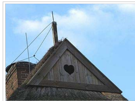
An Eulenloch ("owl-hole") in northern Germany lets barn owls access the attic for nesting
